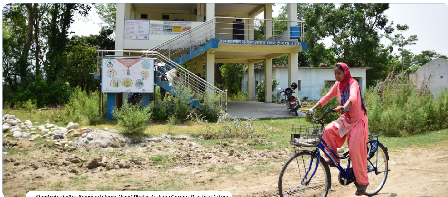
Flood safe shelter, Bangaun Village, Nepal. Photo: Archana Gurung, Practical Action
