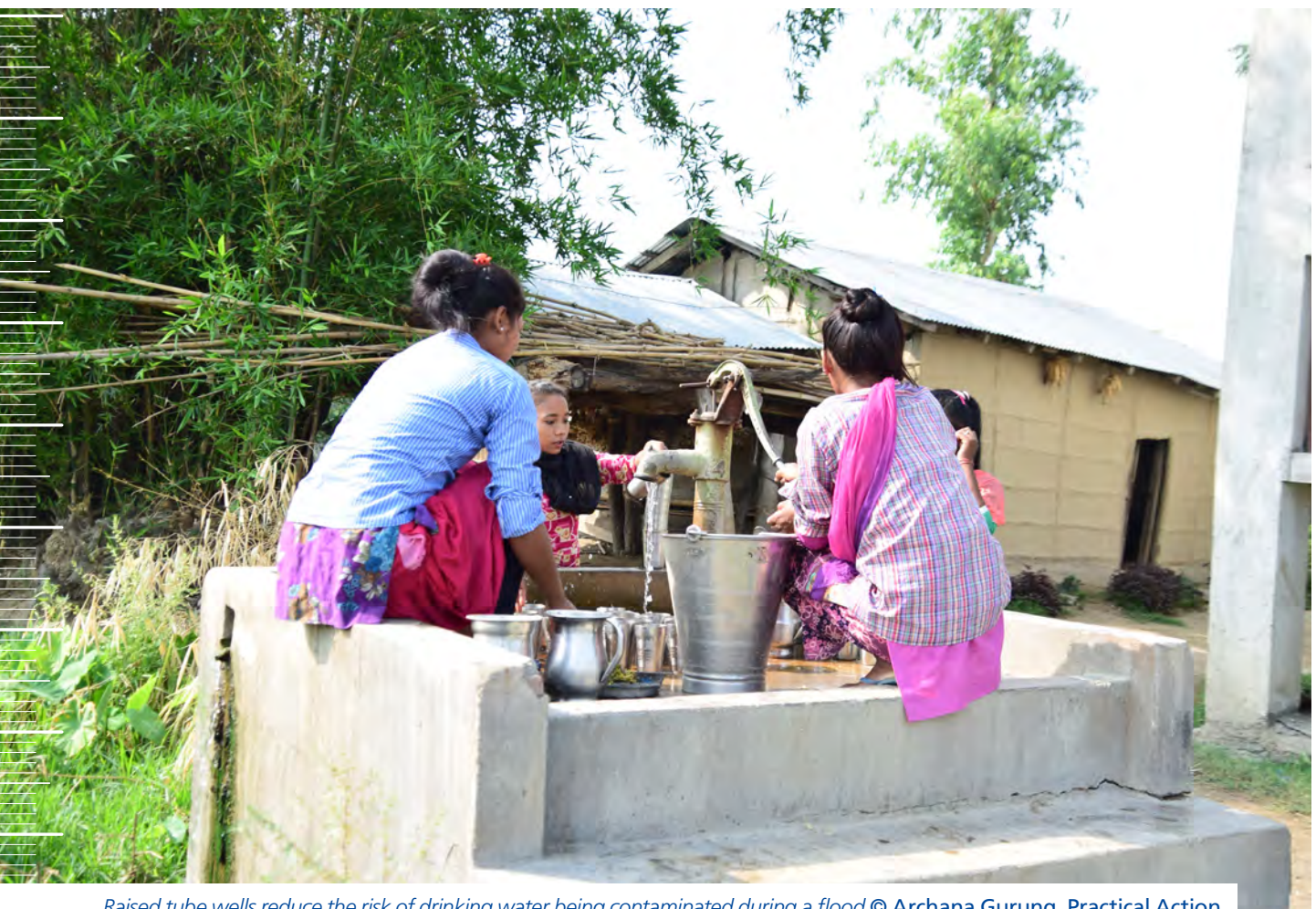
Raised tube wells reduce the risk of drinking water being contaminated during a flood © Archana Gurung, Practical Action
